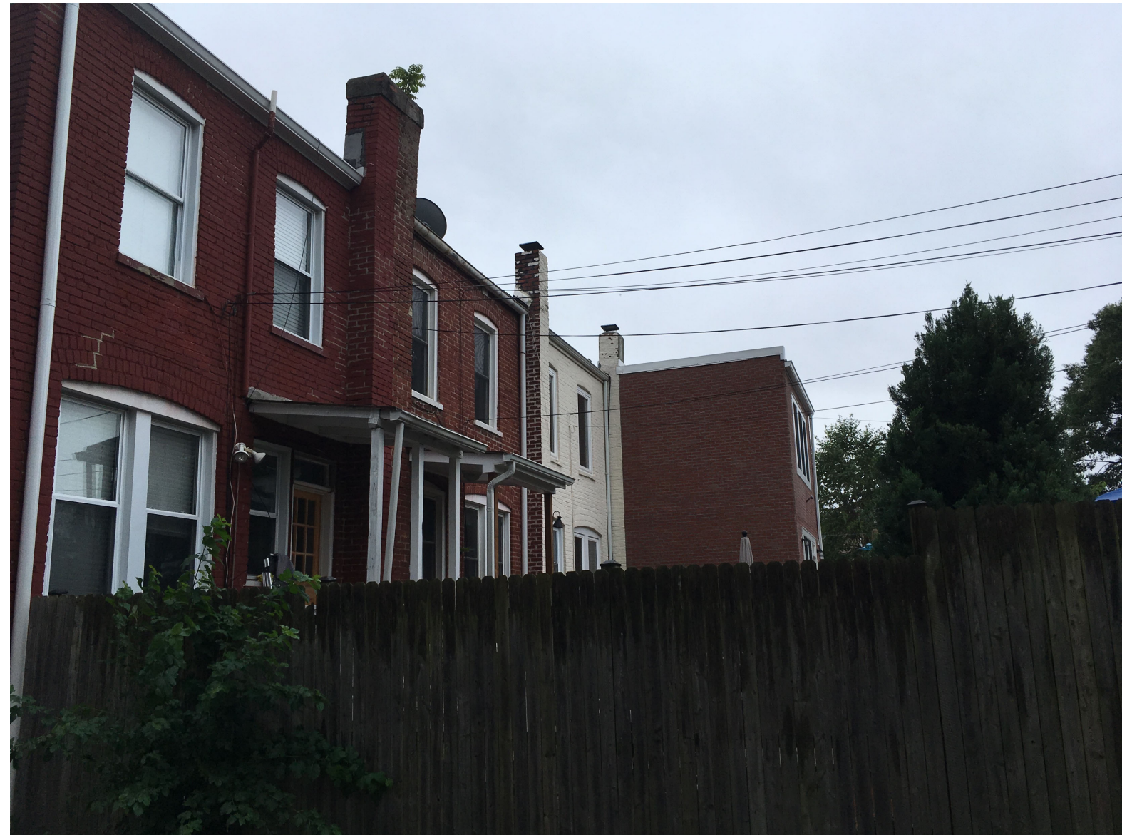
REAR VIEW FROM SIDE ALLEY (LOOKING EAST)
