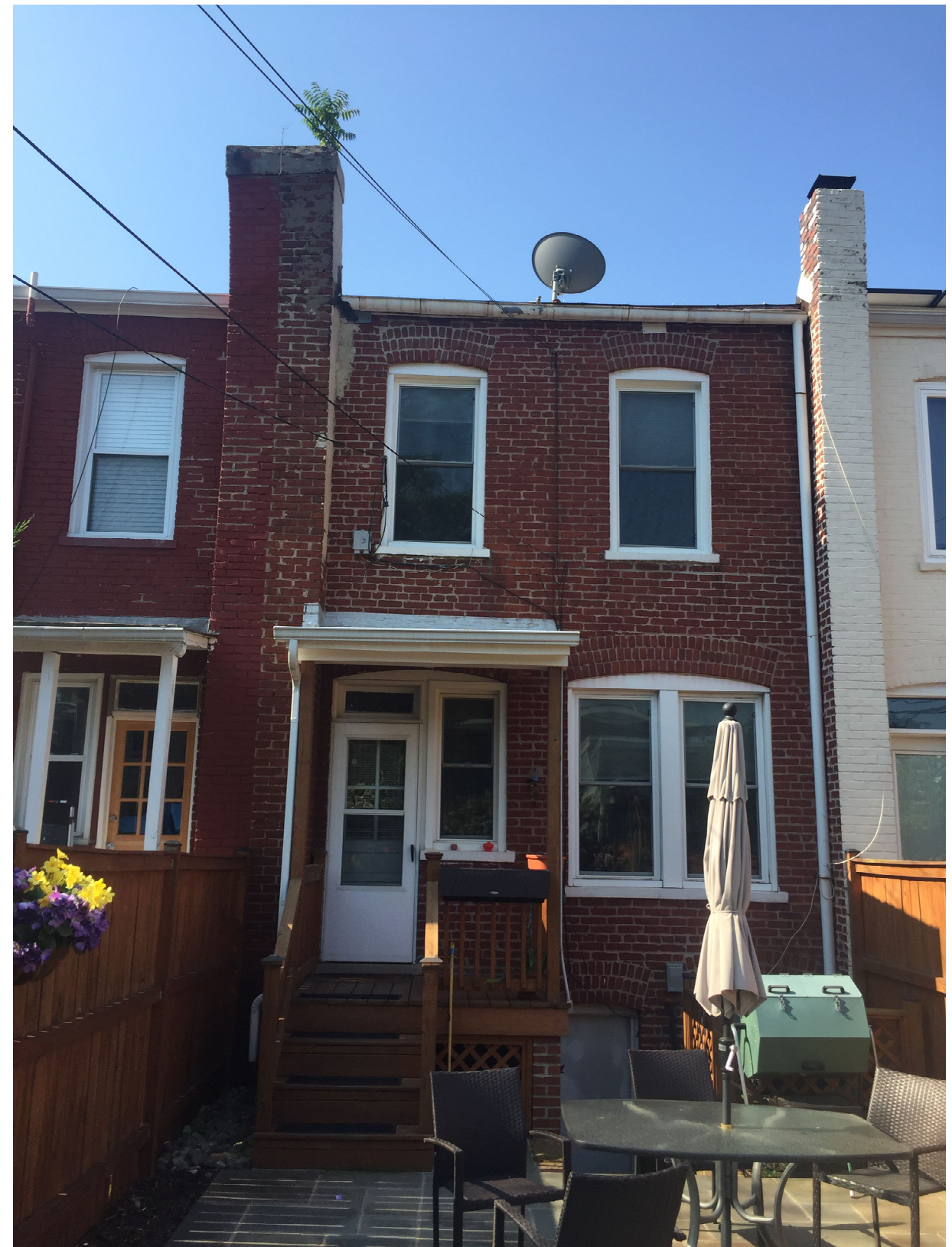
EXISTING REAR FACADE
